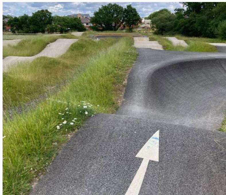
Pump track at Blythe Valley Park, Solihull.
